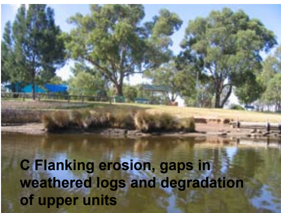
Figure 6.2 Photos of failed log walling
