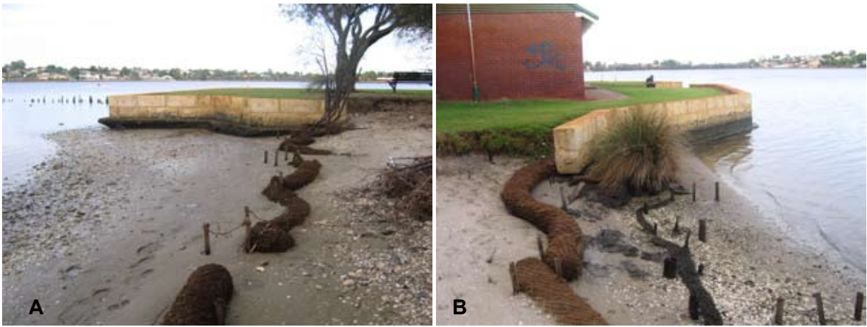
Figure 7.4 Flanking erosion (A – downstream; B – upstream) of cut block walling at Shelley Sailing Club
