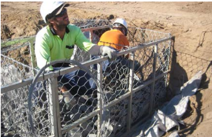
Figure 5.7 Hand placing rock in partially filled gabion unit
