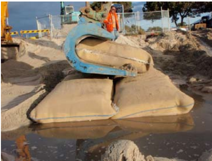
Figure 9.4 Placement of 2.5m 3 geotextile sand container
