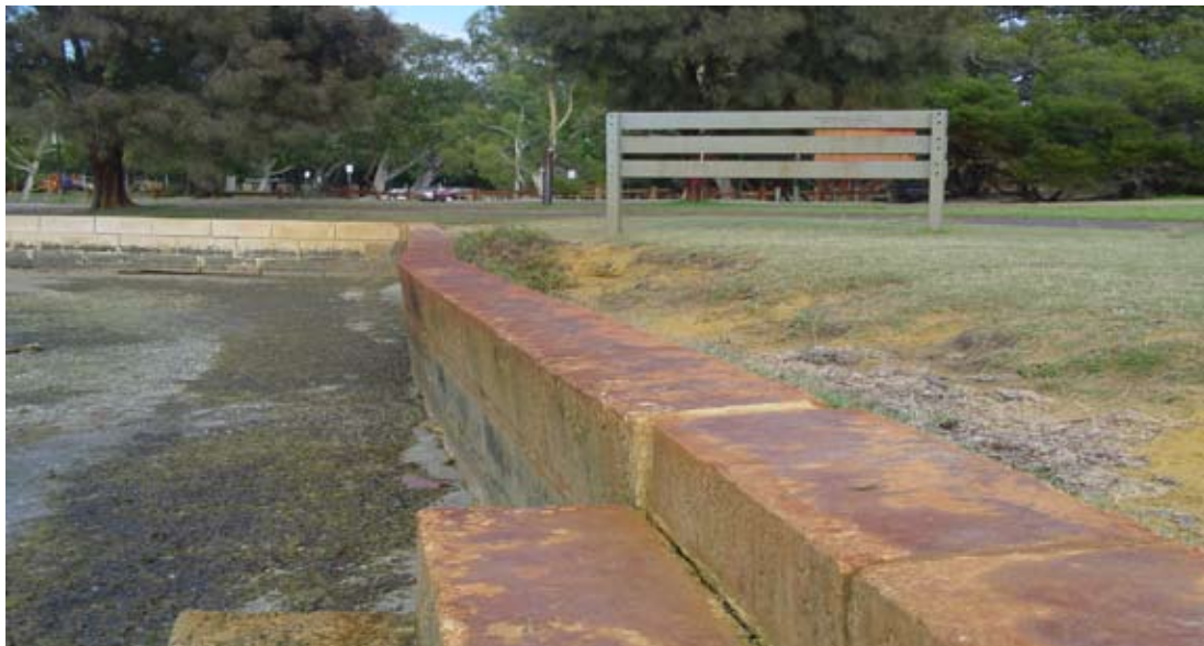
Figure 7.1 Bed elevation lowering in front of a vertical cut block wall – Qantas Boat Ramp
