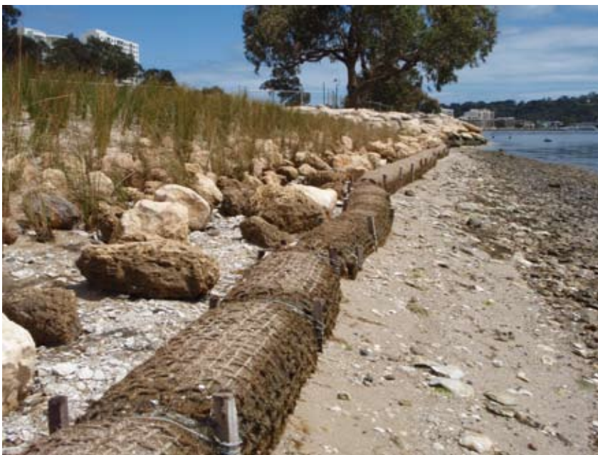
Figure 3.1 Coir logs installed according to best management practice at Sir James Mitchell Park
