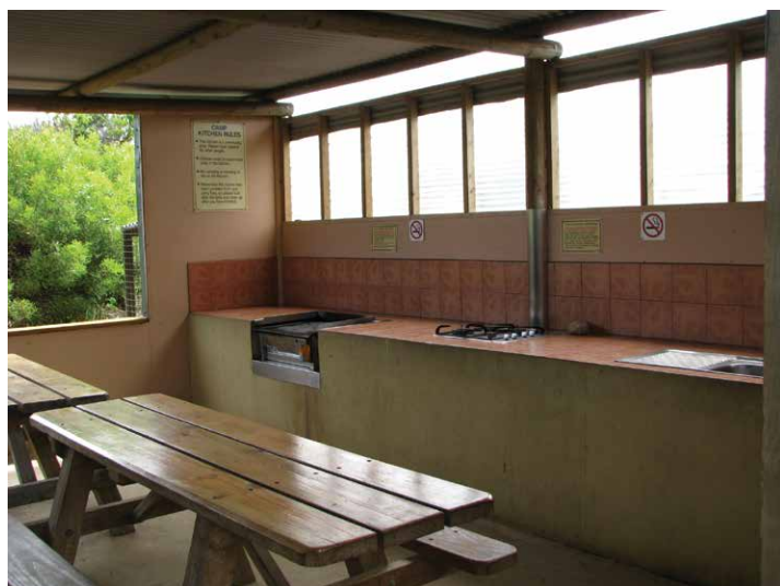
Camp kitchen at Le Grand Beach, Cape Le Grand National Park. Within the recreational site hierarchy, Le Grand camping area is classed as 'high' due to the level of facilities provided and access. Photo - Tegan Laslett
