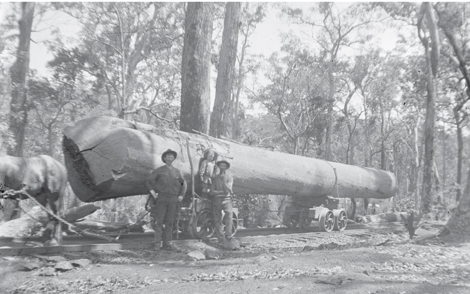
A log is hauled on rails out of the South West forest by horses, probably near Lyalls Mill - State Library of Western Australia -Image
