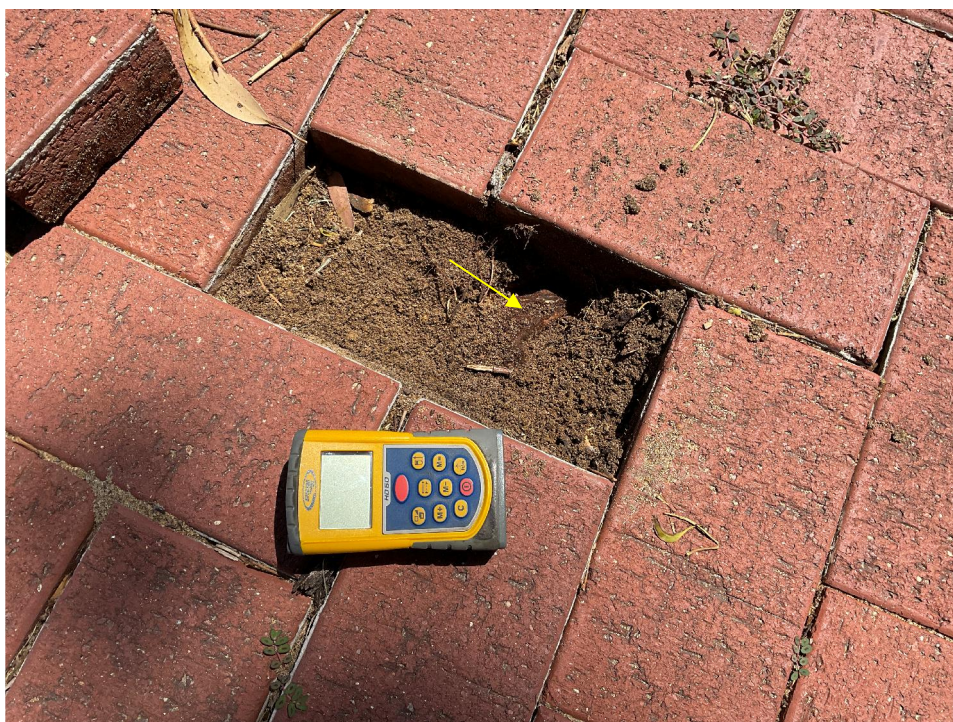
Figure 14. Example of a wounded root section (see arrow) in contact with the underside of displaced pavers, which is larger in diameter than the adjacent non-wounded section of the same root.
