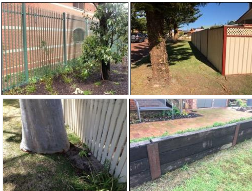
Figure 8. Example of root-sensitive options to span a low wall or fence structure across the root plate of a tree whilst limiting excavation to avoid severing large woody roots: (a) post and palisade fencing; (b) post and panel colorbond fence; (c) timber picket fence; (d) i-beam and sleeper low wall.
