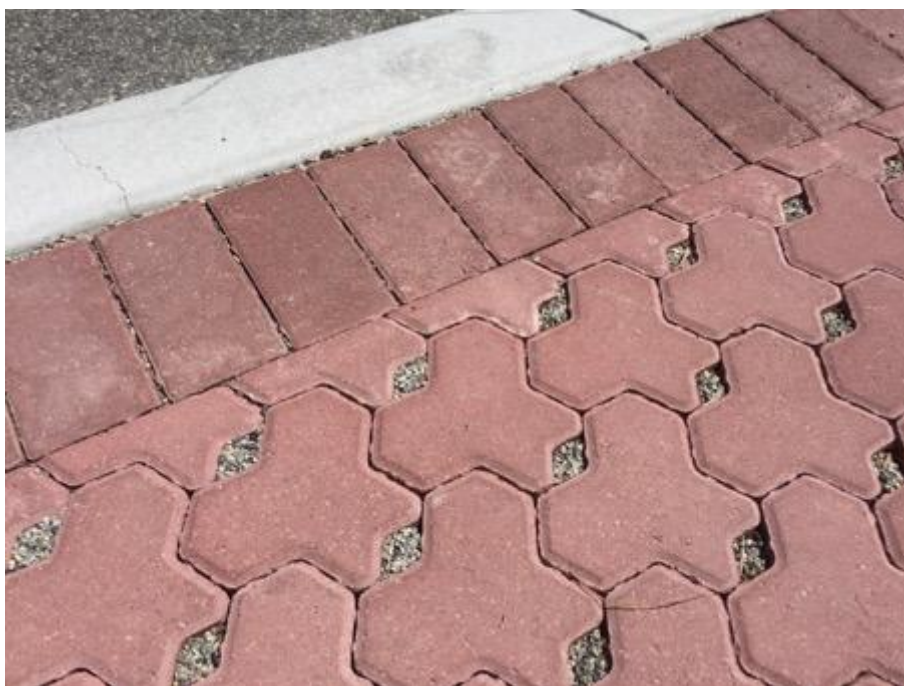
Figure 7. Where hard surfacing is proposed adjacent to existing trees the use of permeable paving provides an option to improve water/ nutrient infiltration and adequate soil aeration (oxygen) to the small absorbing roots – required to maintain healthy trees.
