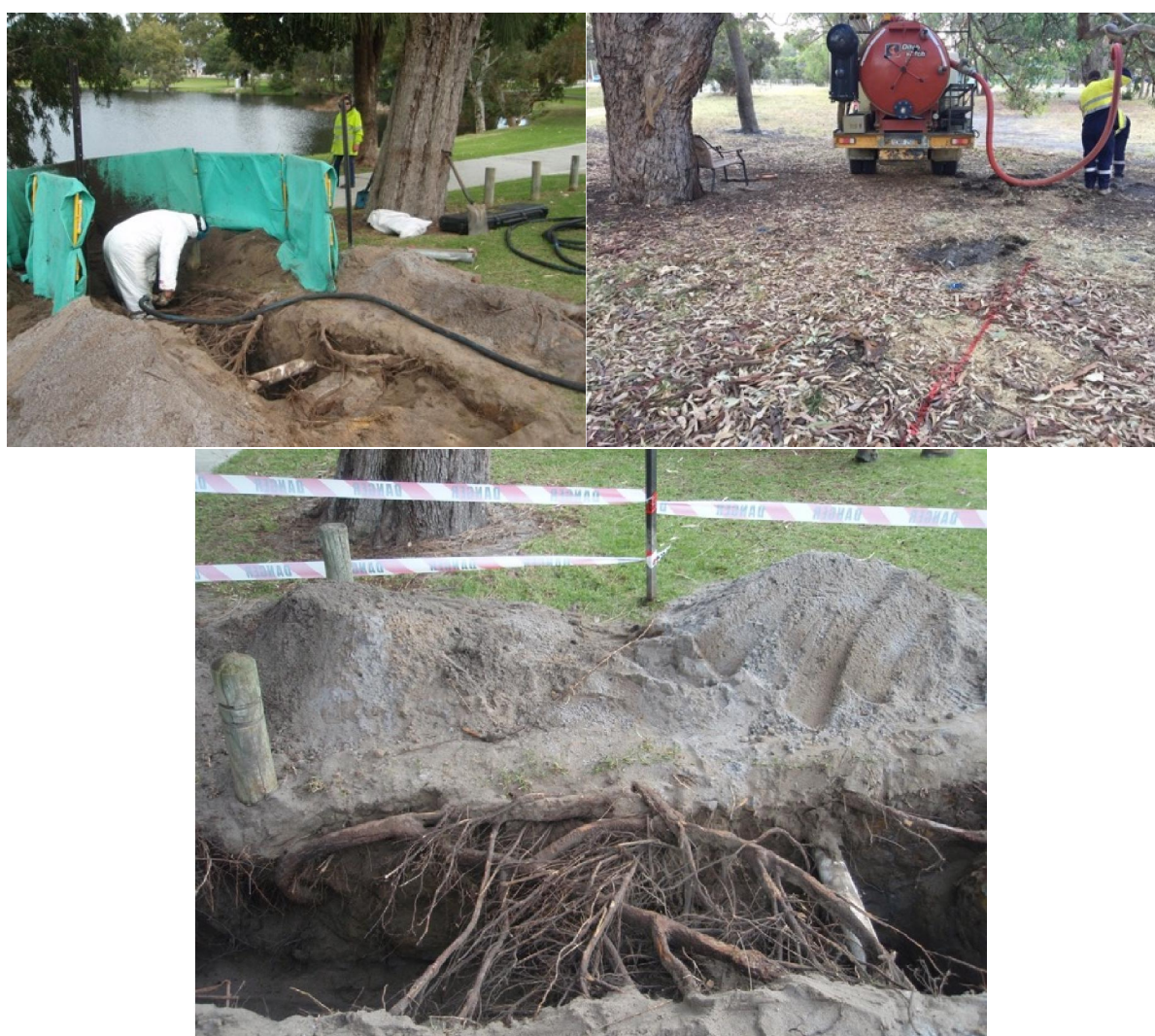
Figure 11, 12 & 13. Example of air-spading and soil vacuum to remove soil within the tree protection zone without damaging or severing tree roots, thereby allowing the installation of below-ground services beneath the rootplate.
