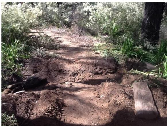
Figure 12: Localised erosion downstream of Mundaring Weir Road.
