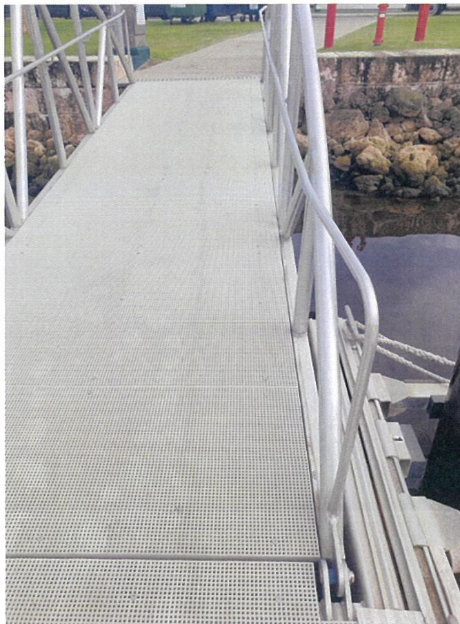
Figure 3: Decking similar to the micromesh proposed for use on Jetty 8
