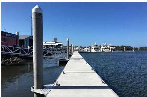
**Figure 4** - Floating concrete pontoons
