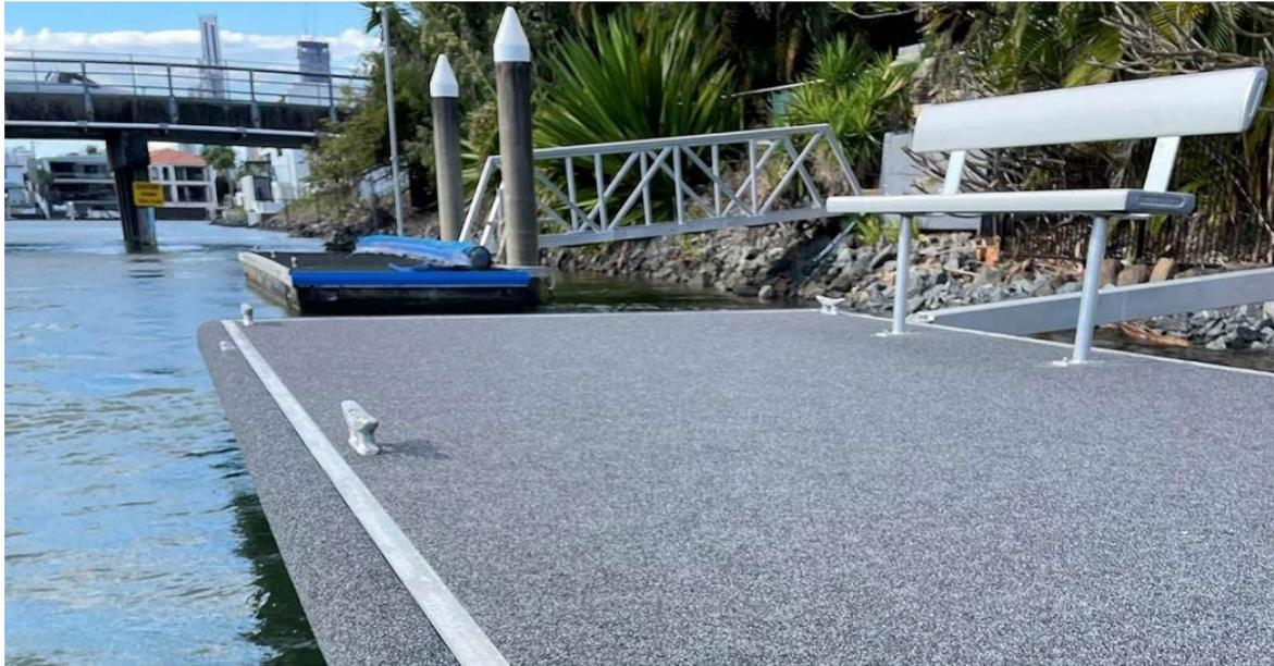
**Figure 3** - Example of a bench seat on a floating pontoon.
