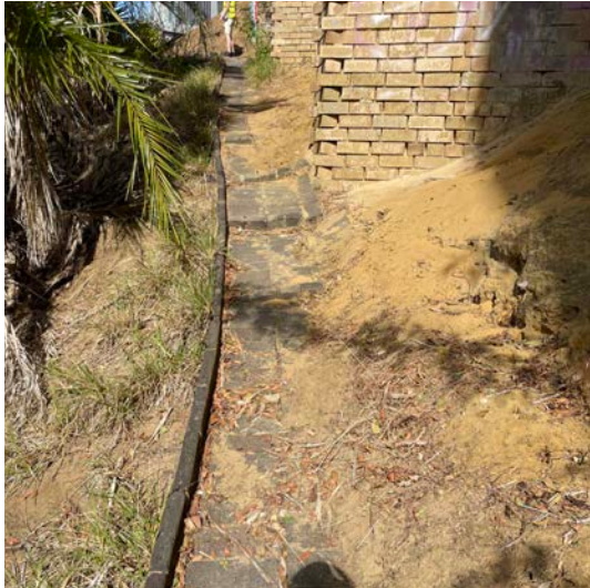
Fig: Undermined walkway and yellow sandy fill
