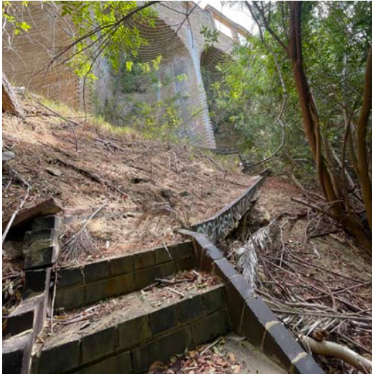
Fig: Brick stair and walkway undermined
