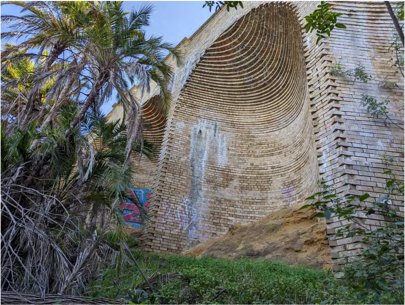
Photograph 3: Arched retaining structure
