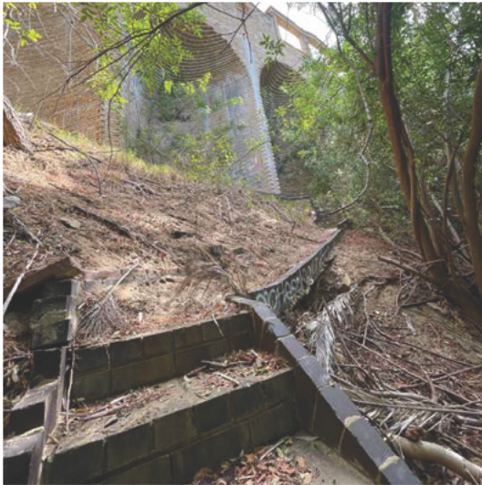
Fig: Brick stair and walkway undermined
