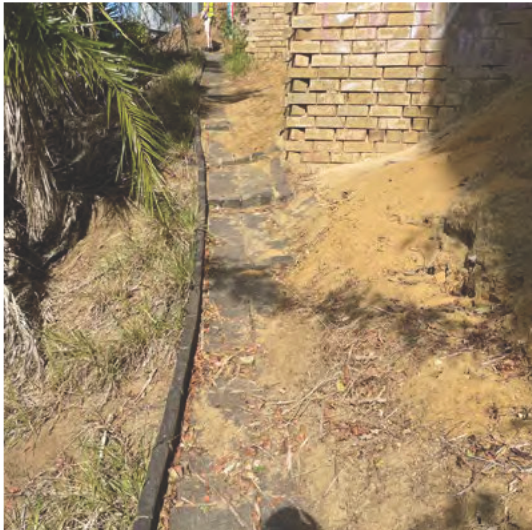
Fig: Undermined walkway and yellow sandy fill
