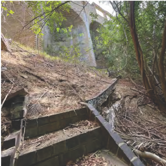
Fig: Brick stair and walkway undermined
