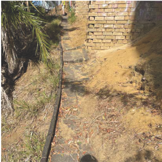
Fig: Undermined walkway and yellow sandy fill
