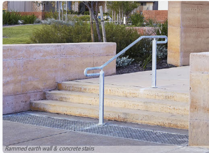
Rammed earth wall & concrete stairs
