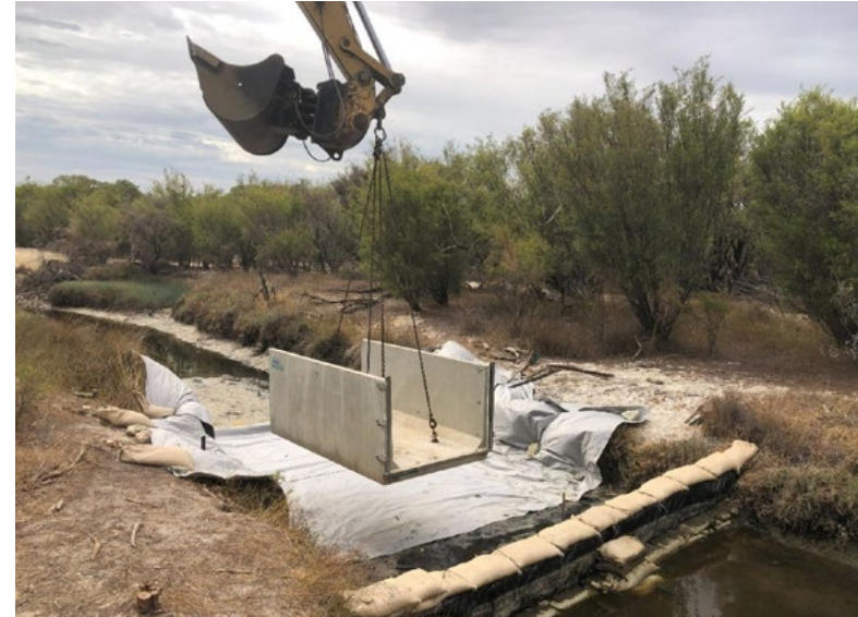
The culvert/stop-board unit was installed over summer when there was no flow in the drain. However, a sandbag wall was required to keep tidal water out of the construction site.
