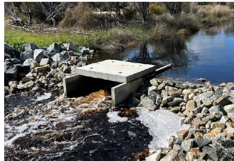
August 2025. With some stop-boards fitted the structure raises the upstream water level. Any excess flow can pass either side of the culvert over the rock sidewalls. Photos - Rick James.
