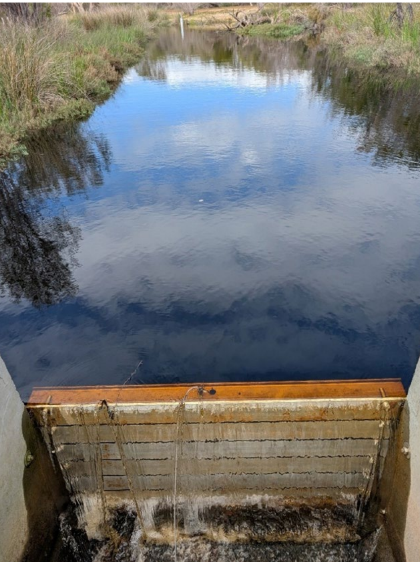
With stop-boards fitted the water level upstream of the structure can be kept high and this helps raise local groundwater levels. Photo - Rick James.
