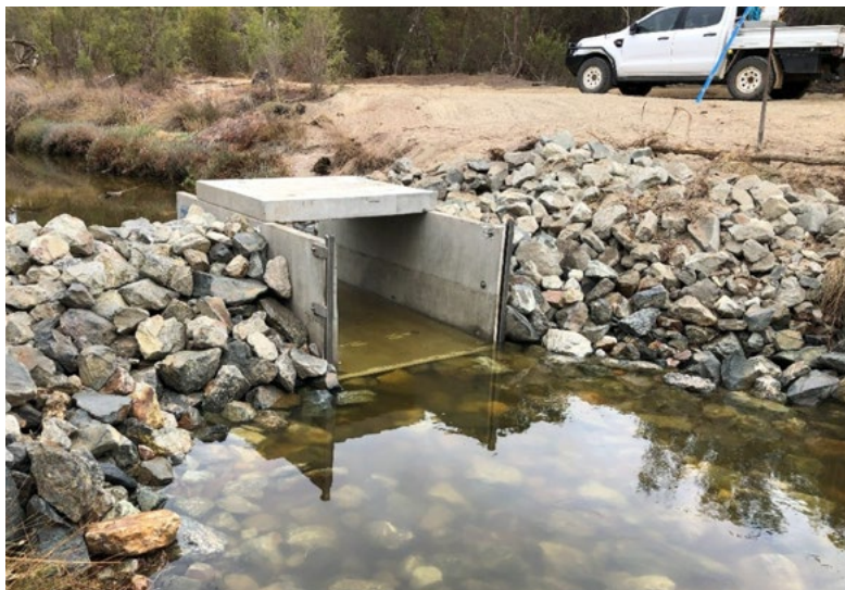
The completed structure in 2024 (view looking downstream). The rock was carefully placed against the plywood/plastic/geofabric sidewalls. This arrangement prevents water flowing through the rock meaning that all flow must go through the culvert, or over the top of the rock walls.
