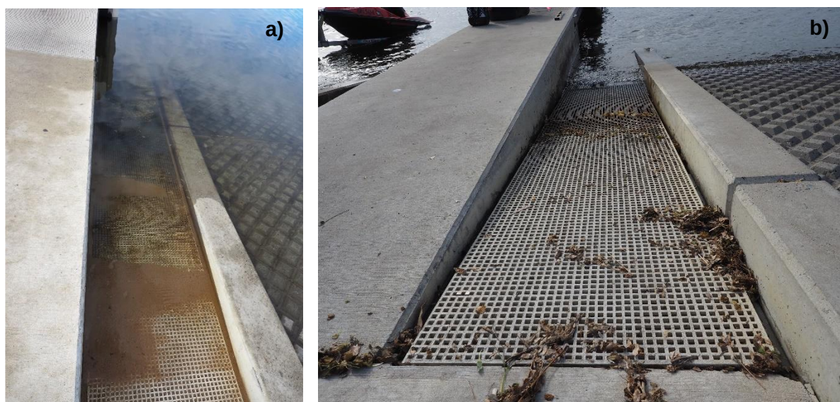
Figure 34. Examples of fibre reinforced plastic exposed to wet and dry cycling at Deep Water Point (a) and Point Walter boat ramps (b).
