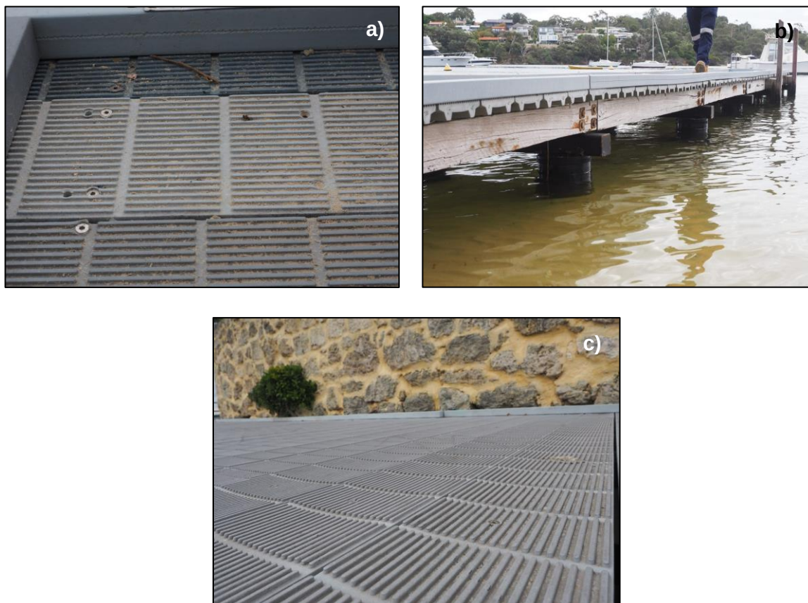
Figure 21. Deformation of recycled plastic decking observed at Pollard Park jetty (a, b) and Applecross boardwalk (c).
