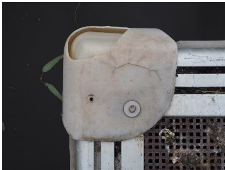
Figure 31. Damaged rigid capping used on corners of the pontoon at Middle Swan Reserve.
