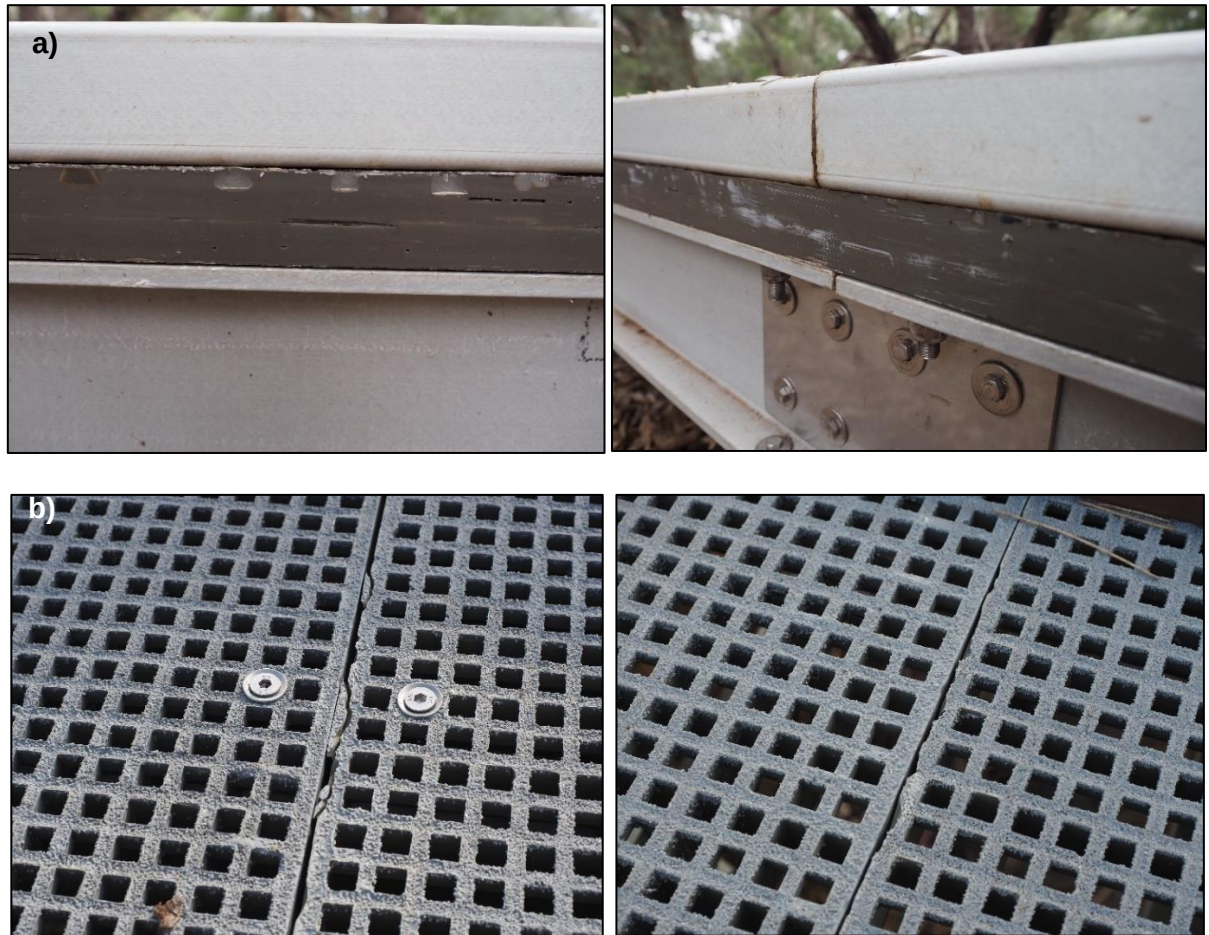
Figure 18. (a) Fibre reinforced plastic (FRP) kick rail (top), FRP mini mesh edging (middle dark grey layer) and FRP substructure (bottom layer) along board walk at Thornlie nature reserve; (b) FRP decking joints at Melville bird view platform.
