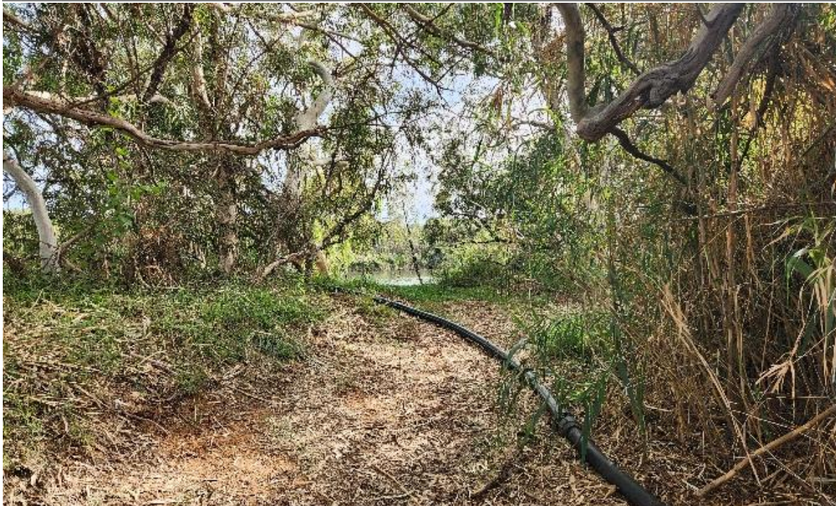
Above: Section of private pipeline through Jiggabiddi Nature Reserve. Photo Veronica Newbury/DBCA
