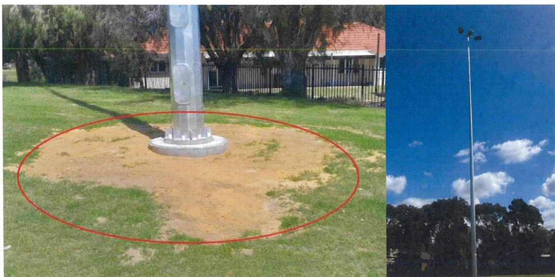
Figure 3: Two photos showing examples of poles, similar to what will be installed at Charles Court Reserve – left: pole base and above-ground portion of footing; right: top of a pole with three floodlights.
