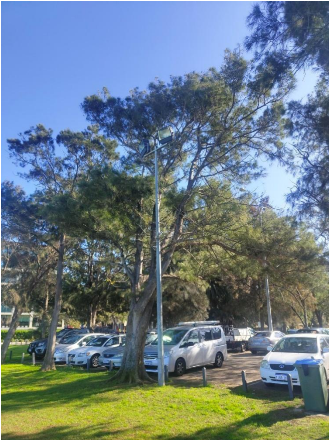
Northern side of reserve at the rugby clubroom carpark, existing light tower (10m high).
