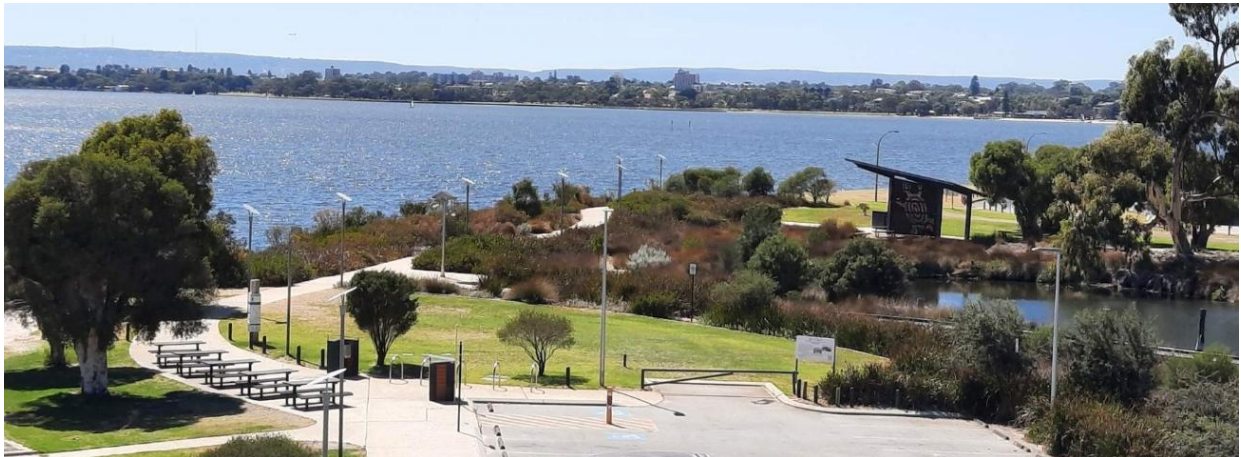
Figure 6: View from Narrows Bridge across the carpark and the adjacent lease area, showing existing vegetation within the lease area (grass, sedges and shrubs) and surrounding area.
