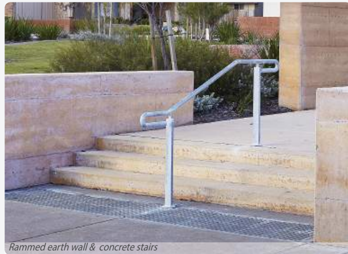
Rammed earth wall & concrete stairs
