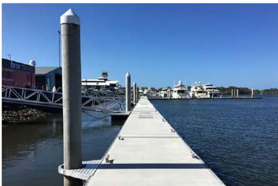
Figure 4 - Floating concrete pontoons
