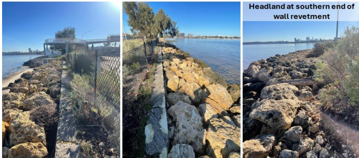
Figure 4-9: Thelma Street to north of Cale Street – Rock Revetment and Headland
