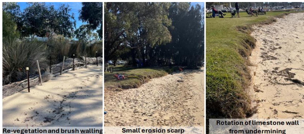
Figure 4-7: Erosion at the Pelican Point Sea Scout Group
