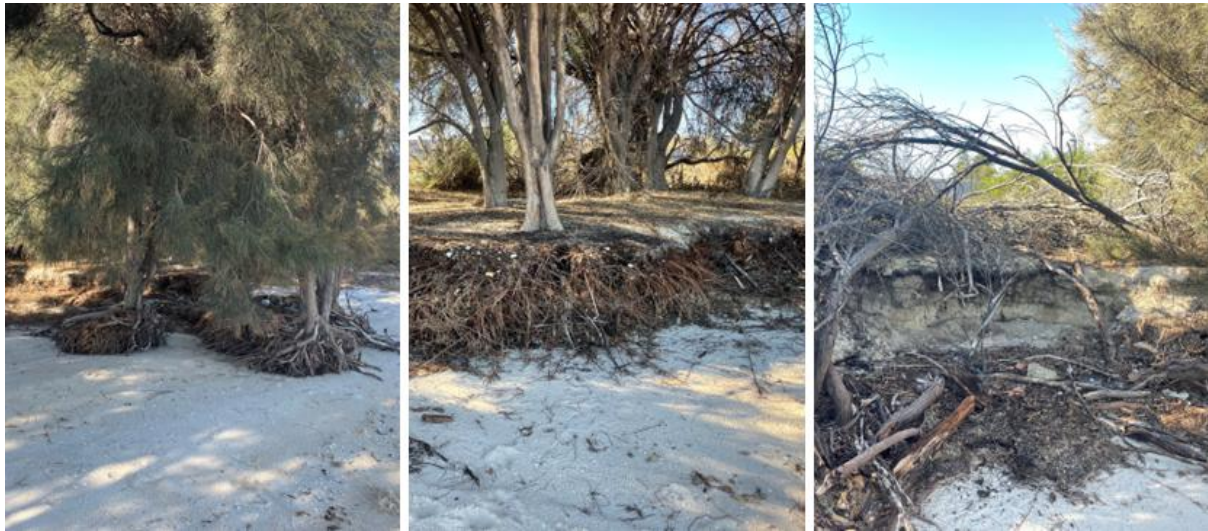
Figure 4-10: Erosion Scarps and Tree Loss and Undermining Near Cale Street
