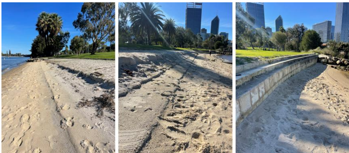
Figure 4-2: Southern Segment – Beach with Headland Controls
