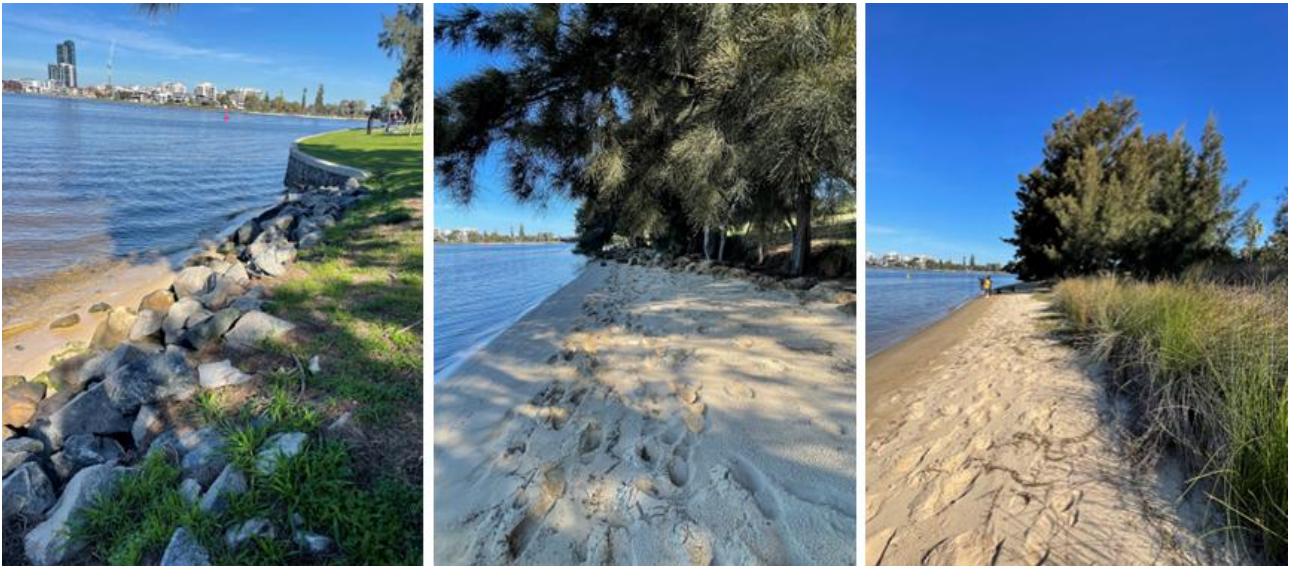
Figure 4-3: Northern Segment – Vegetation and Rock Toe Protection
