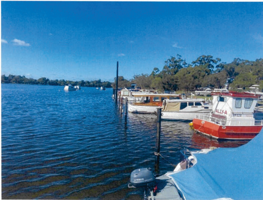
Figure 6: Looking across the jetty at the southern area of the facilities (photo taken in 2025)
