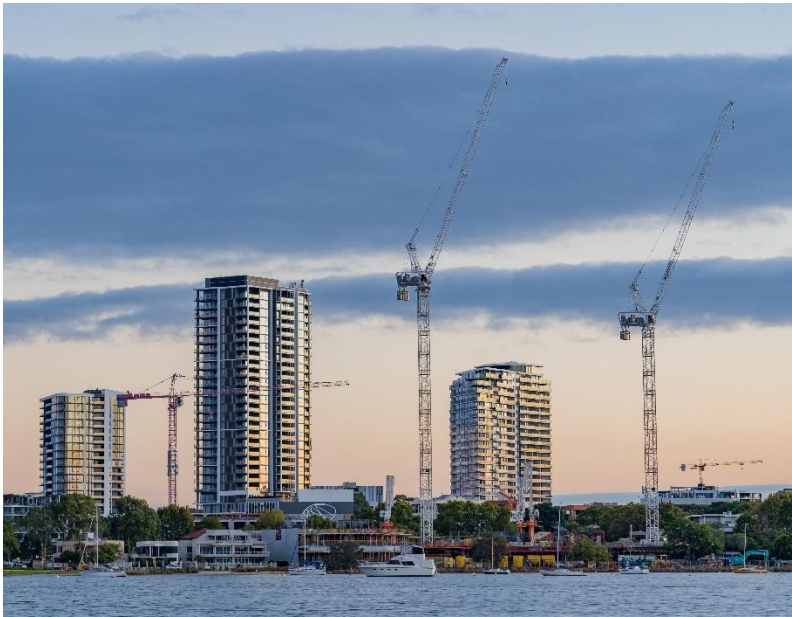
Construction of Canning Bridge apartments. Photo – Peter Howie, Department of Biodiversity, Conservation and Attractions
